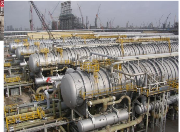
MED Facility Erection, Reliance, India
