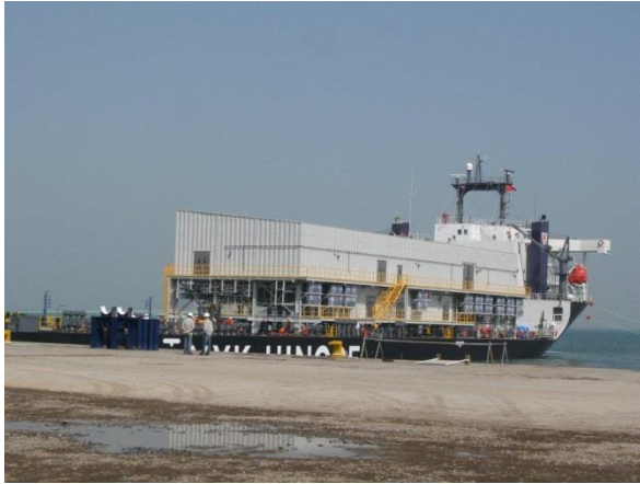
Prefabricated RO Plant 140K m3/day Cape-Preston, Australia
