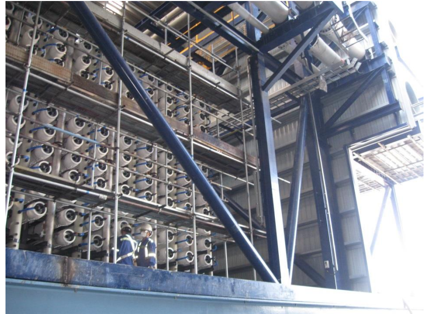
SWRO Skid Installed within Membrane Building Module and Pressure Vessels Installed
