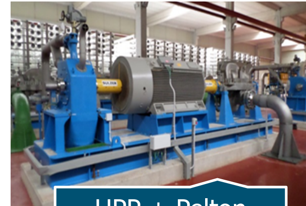
HPP + Pelton Turbine 1 st Stage
