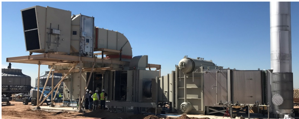
6.5 MW Natural Gas CHP
