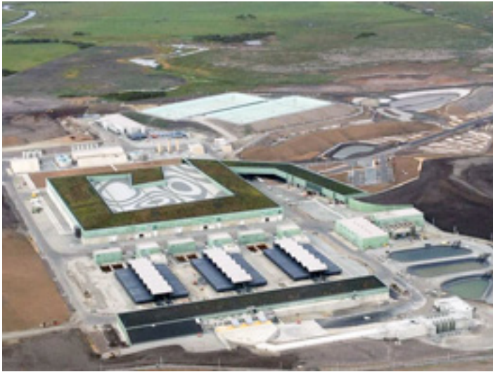
450,000 m 3 /d Victorian Desalination Plant – Wonthaggi, Australia
