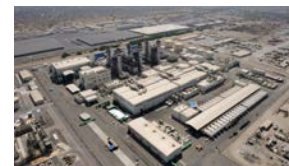
Barka 2 (Oman) - BOO Desalination – 136 mld
