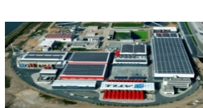
Barcelona (Spain) - DBO Desalination – 200 mld
