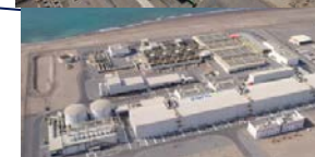
Barka 4 (Oman) - BOO Desalination – 280 mld
